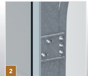
2 Tracks fastened to the opening frame with screws
